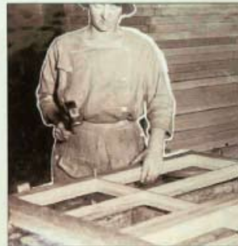
A woman in the construction trades, "pinning in sash" on a window (1919).
