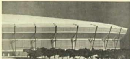
The "Domed Stadium" is on schedule and the oval is nearly complete. In approximately a year, the first Twins game will be played in the dome. (Special thanks to Howard N. Kaplan, CHNK Architectural Photography for use of this photo.) (Photo submitted by Local 292, Minneapolis, Minn.)
