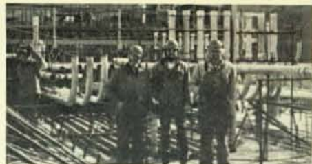
On the job at Phipps Bend Nuclear Plant, John McLain, Walter Quiggle, and Bob Chestnut of Local 934, Kingsport, Tenn., stand before a rack of four- and five-inch conduit. (Photo by Dennis Cornwell)
