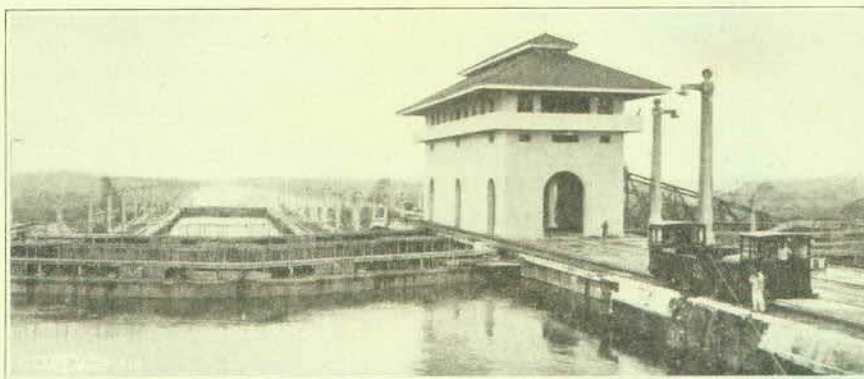
CONTROL HOUSE, GATUN LOCKS. ATLANTIC ENTRANCE IN THE DISTANCE.
