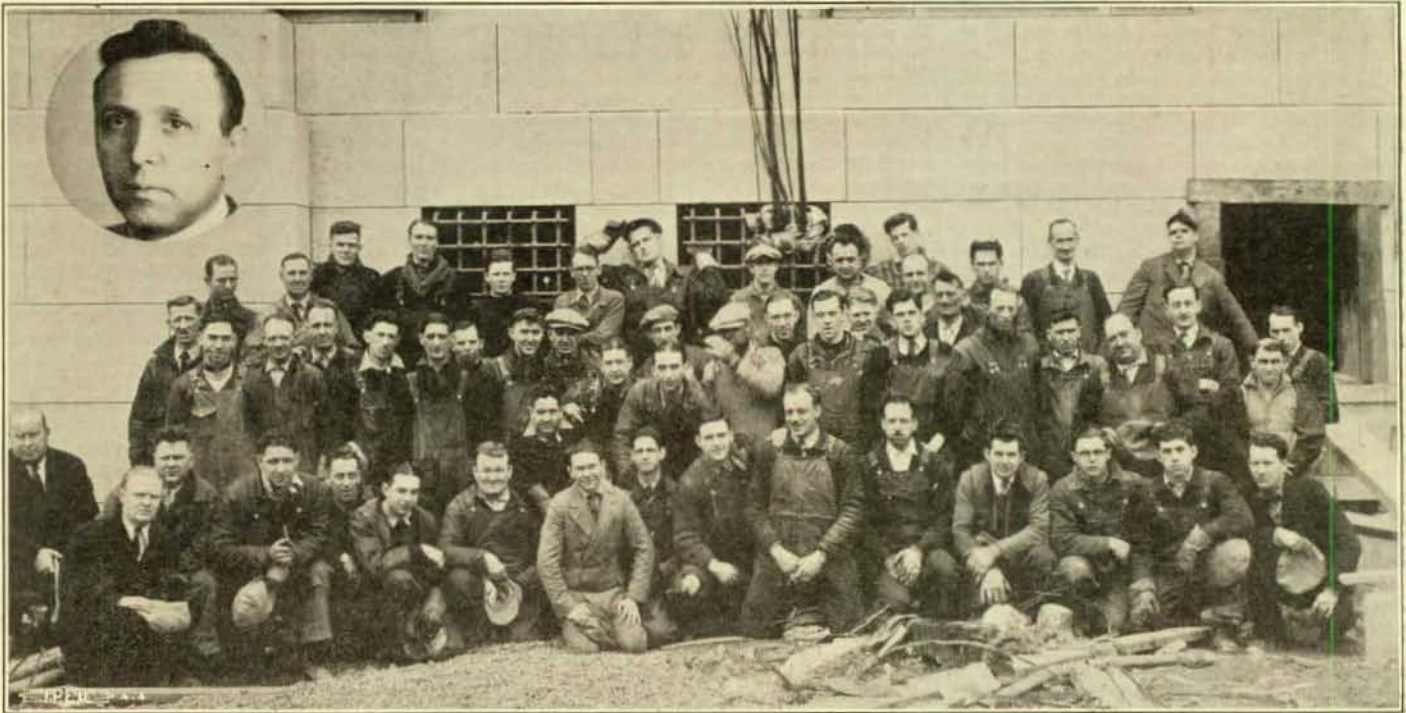
THE 32-STORY NEW YORK STATE BUILDING IS BEING WIRED BY THIS CREW FROM L. U. NO. 696, ALBANY.
