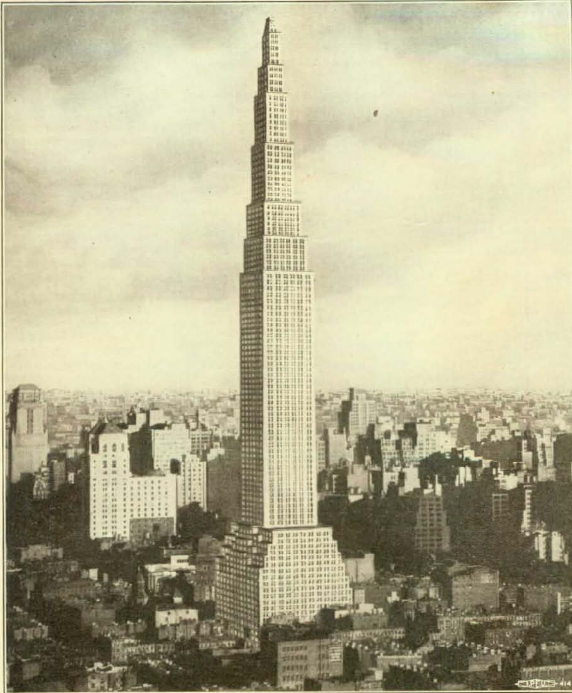
PROPOSED LARKIN TOWER, NEW YORK, 108 STORIES HIGH—AN INNOVATION IN THE METROPOLIS OF ARCHITECTURAL WONDERS.
