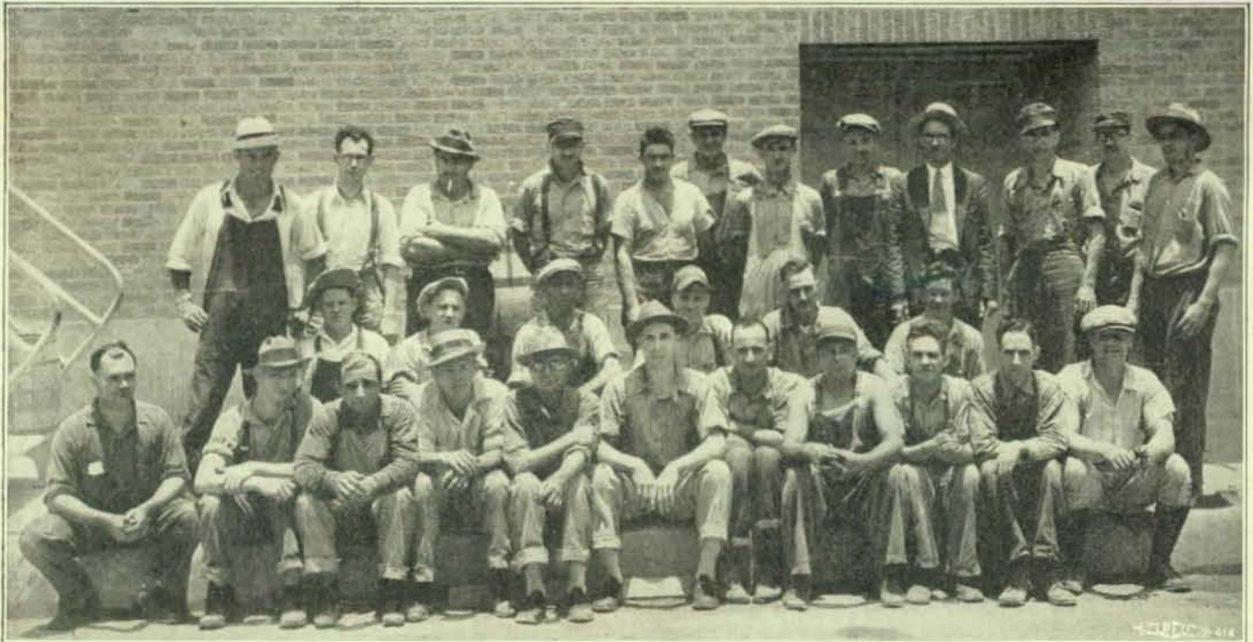
THIS FINE CREW WIRED THE GREATER MAJESTIC THEATRE BUILDING (See Frontispiece). ALL MEMBERS OF LOCAL UNION 60, THROUGH THE COURTESY OF BROTHER DEHART. BROTHER DAVE KRISCH WAS FOREMAN ON THIS JOB.
