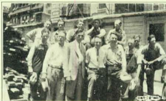
CREW OF L. U. NO. 1141 WHO DID THE WIRING
