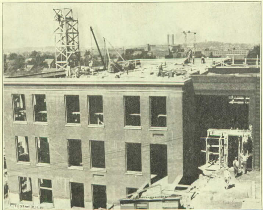
L. U. No. 306 members working on the new wing for the engineering department of the University of Akron.
