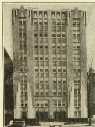
Here is an apartment building in Milwaukee also "skeletonized" with modern wiring.
