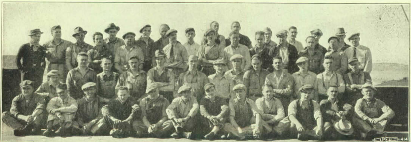
These members of L. U. No. B-569 made new friends for organized labor by the excellence of their power station construction for the San Diego Consolidated Gas and Electric Co.
