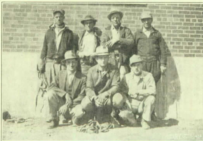
The crew which did the outside electrical work for the white housing project in Nashville, members of L. U. No. 429.
