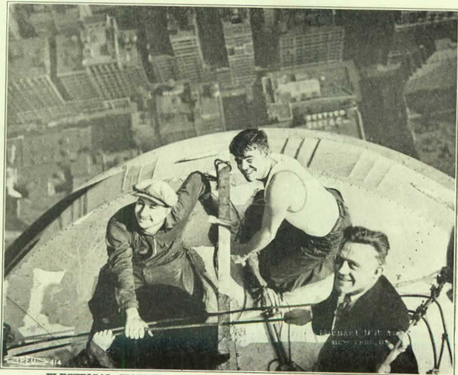
ELECTRICAL WORKERS OFTEN WORK IN HAZARDOUS POSITIONS
