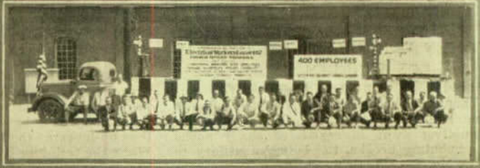
Utility workers of I. U. 607 with a huge float boasting electric power
