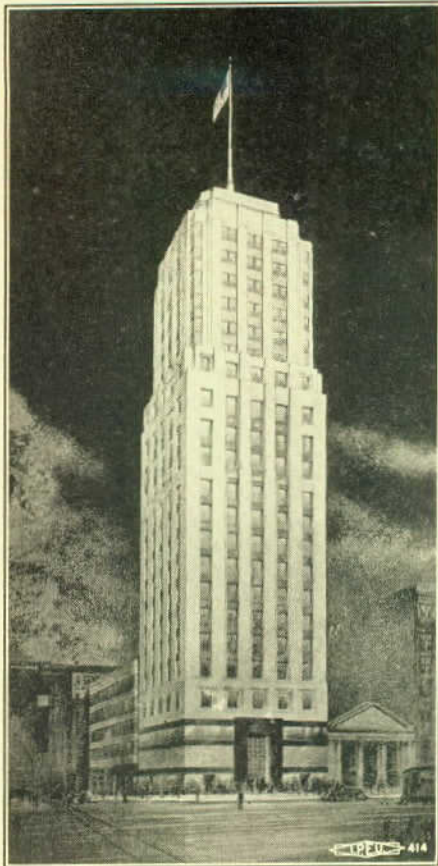
Central Tower, San Francisco, is headquarters for electrical workers on Pacific Coast.
