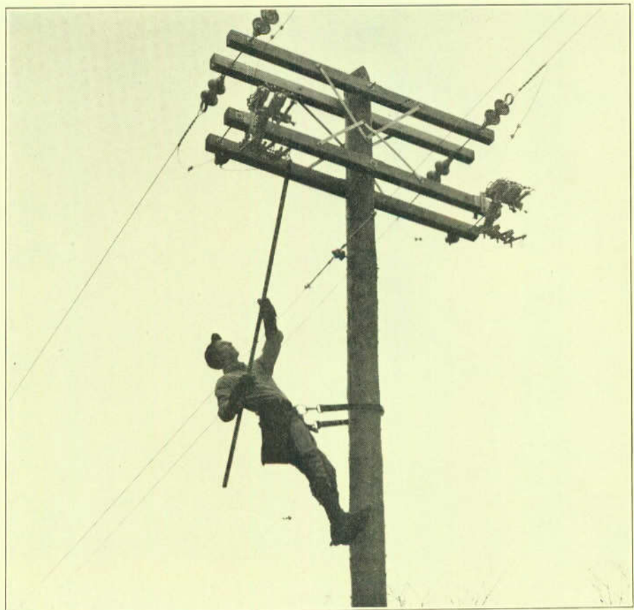
LINEMAN AT WORK
