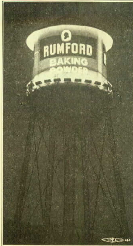
A striking display, the first application of fluorescent lighting to outdoor advertising, as installed and reported by L. U. No. 99.
