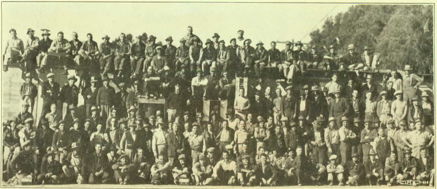
ELECTRICAL CREW OF CAMP SAN LUIS OBISPO, CALIF., TAKEN AT THE ELECTRICAL WAREHOUSE
