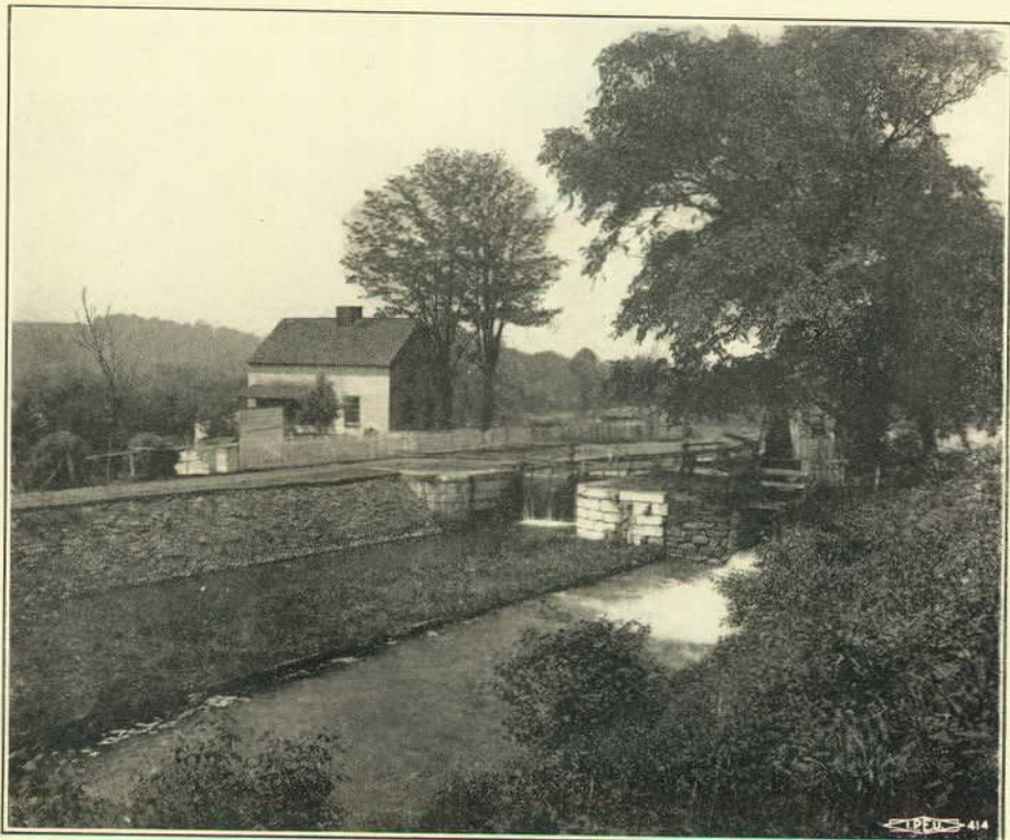
A LOCK AND LOCK HOUSE ON THE OLD C. AND O. CANAL
