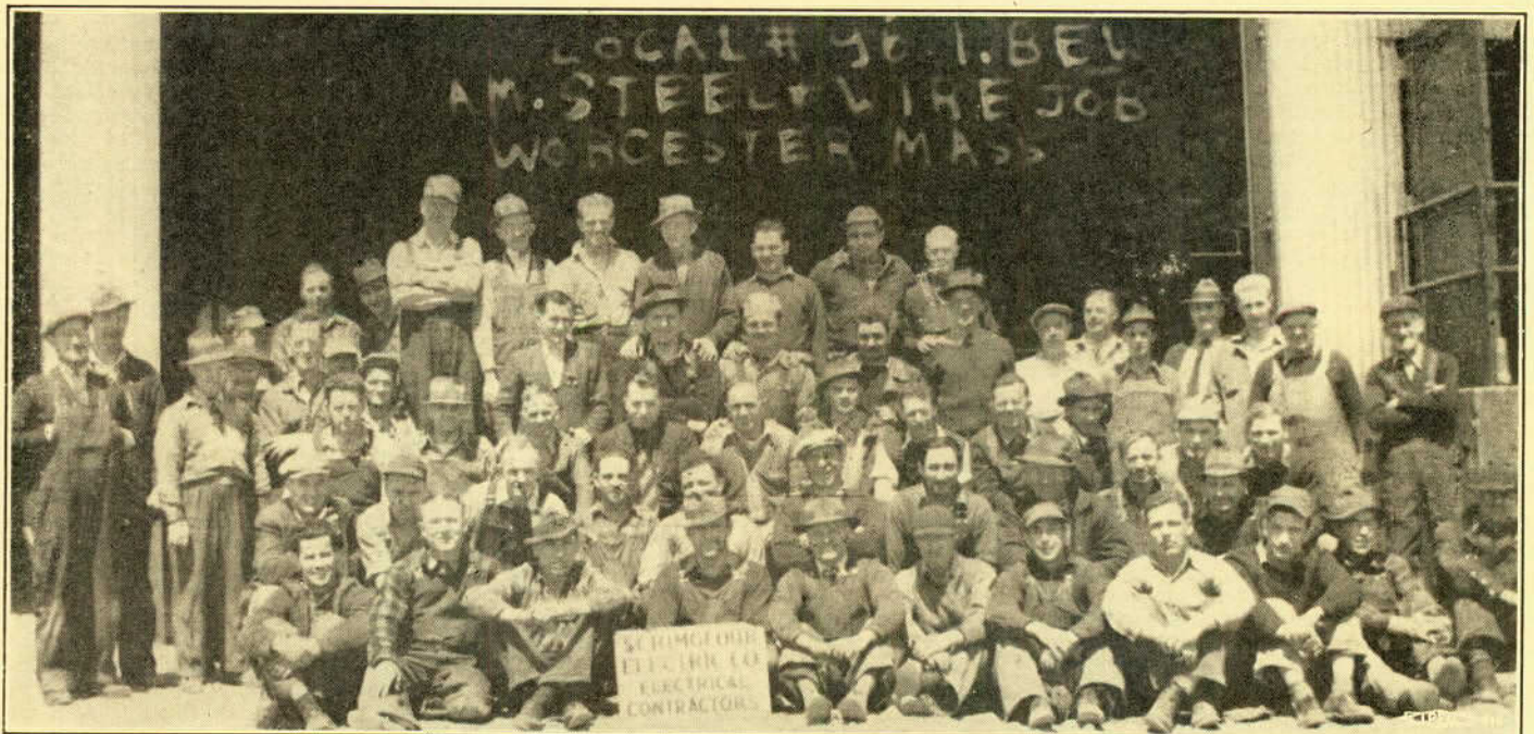
THE LOCAL NO. 96 CREW ON THE AMERICAN STEEL AND WIRE CO. JOB
