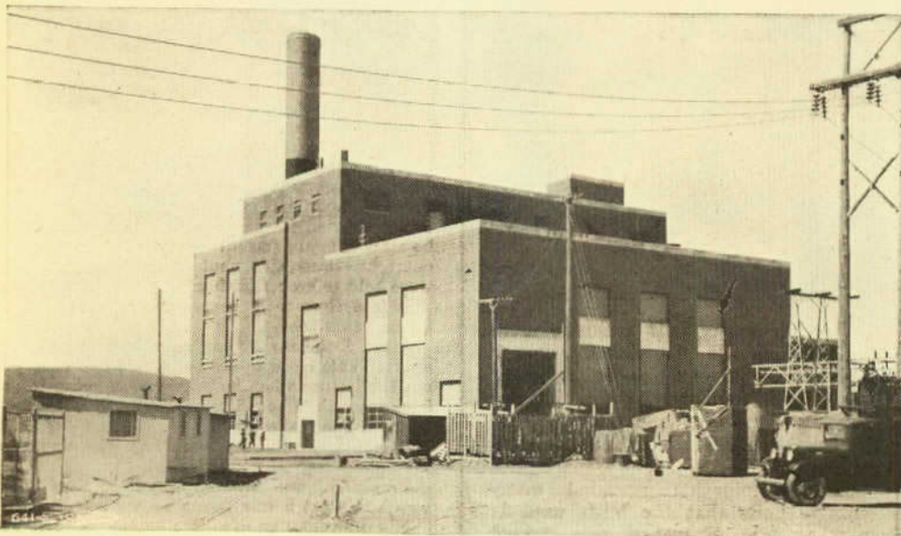
Recently-completed power plant of the New York State Gas and Electric Company described in letter from L. U. No. 325.
