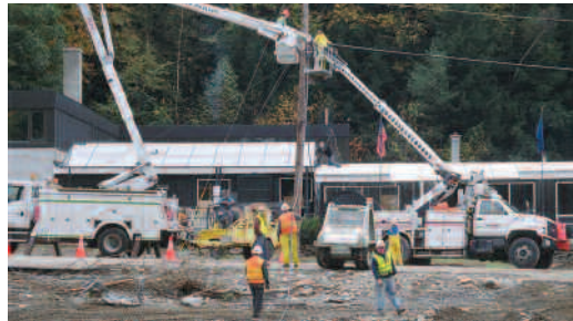
IBEW Local 2320, Manchester, NH, members were lauded for their work restoring vital telecom links after a mas- sive flood.
