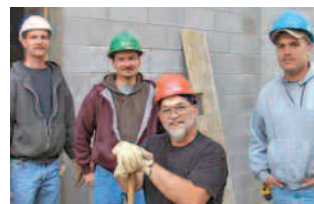
Supporting school bonds has resulted in jobs in Local 557's jurisdiction. Pictured at the new Loomis Elementary School jobsite, from left: Brian Chiesla, Charlie Trumble, Tim Iles and Glen Cooper.
