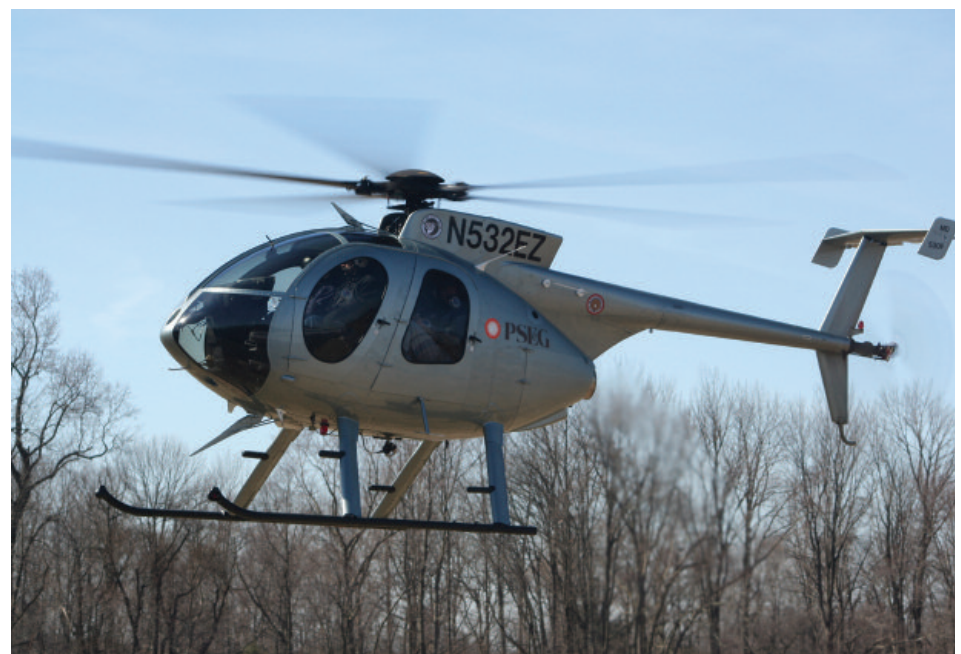
Cranbury, N.J. Local 94 member Eric Carroll pilots PSE&G's first custom-built helicopter for live line repair.
