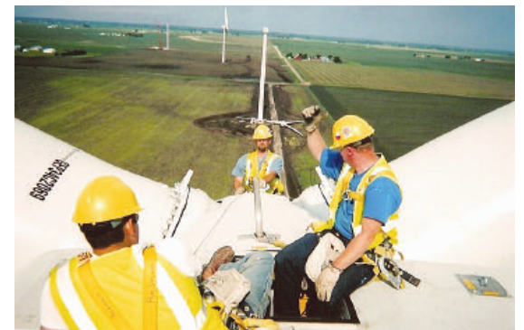
Des Moines, Iowa, Local 347 members Tyler Knoll, left, Ron Cook and Brian Vinke wire a wind turbine hub in Carroll.
