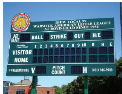
IBEW Local 99 in Providence, RI, installed a state-of-the-art scoreboard for the Warwick American Little League.
