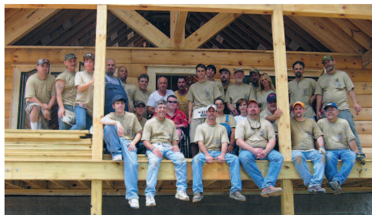
Nashville, Tenn., Local 429 members donated labor to wire a wounded warrior's new home.
