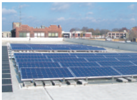
Local 306 members installed rooftop solar array at the University of Akron.
