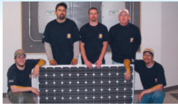
Local 490 graduates and instructor install solar panels: Brain Dean (left), Scott Huot, Jason Strong, Instructor Jim Casey and Steve Reynolds.
