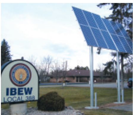
Local 388 installed a new photovoltaic solar array at the union hall.
