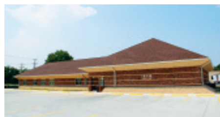
Local 649's new union hall and training center.
