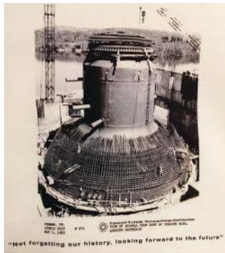
A view of Vermont Yankee Nuclear Power Plant in 1969 shows construction of the drywell.
