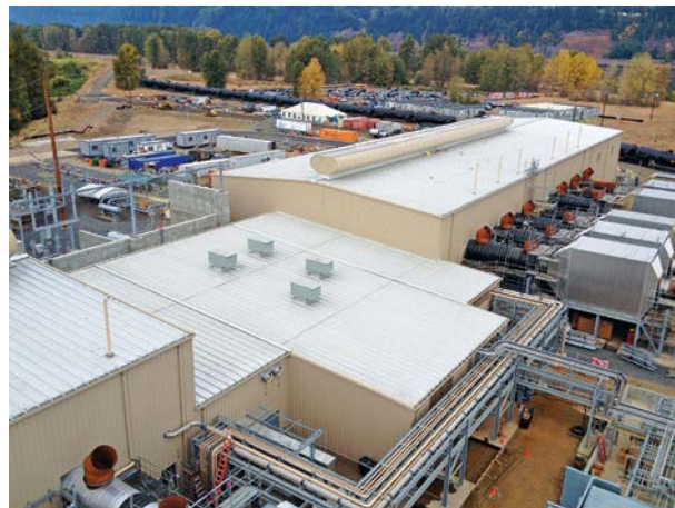
Port Westward Unit 2 facility jobsite for Local 48 project.
