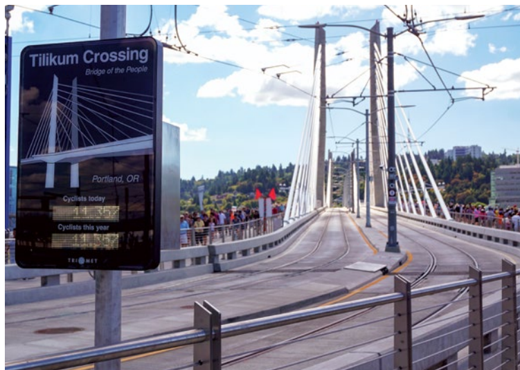
The IBEW-wired Tilikum Crossing connects East and West Portland for pedestrians, bikers, and mass transit users, but leave your cars at home.
