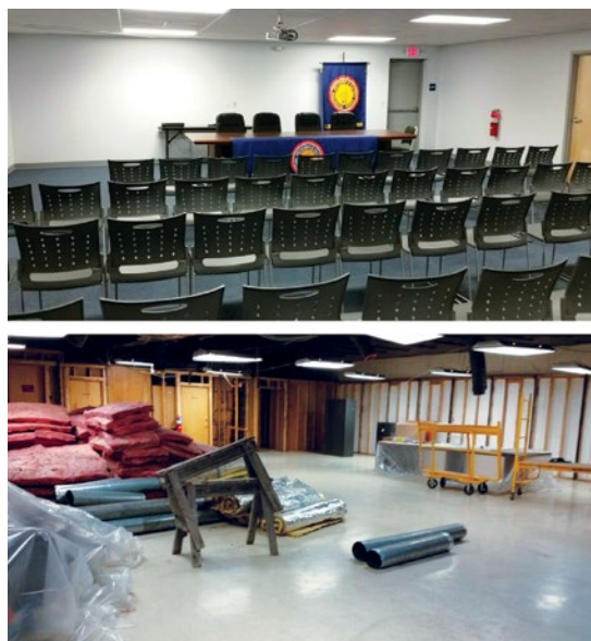
Before and after views of Local 459 meeting room renovation.
