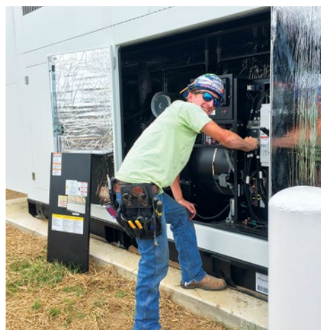
Local 257 apprentice wireman Kyle Schlotz on the jobsite.
