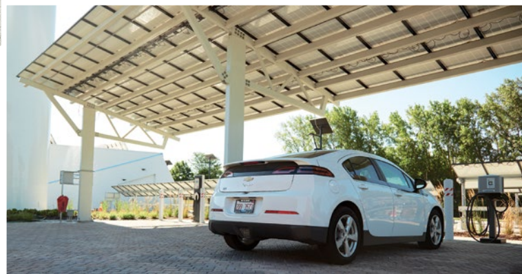
Local 134 and NECA Chicago's new facility provides hands-on training with solar arrays, a wind turbine and even a place to charge electric cars.
