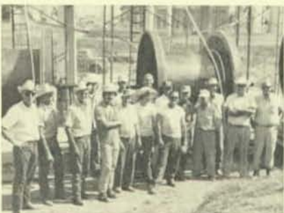
The same crew with Joe De La Campa, project manager.
