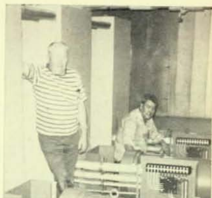
Brothers Red Sundborg, standing, and Bill Hammond, members of Local 100, Fresno, Calif., are shown working on a motor generator at the IRS Building.
