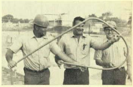
Local 295 wiremen employed by Fagan Electric Company on the new $4-million Trice High School at Pine Bluff, Ark., left to right, are Lee Watson, George Salley, and Jim Wilson.
