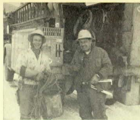
Leonard Cantin, left, and Dan Daley work on a job for Lyndonville Electric.
