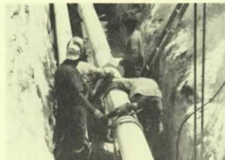
The line is welded together before it is set permanently.
