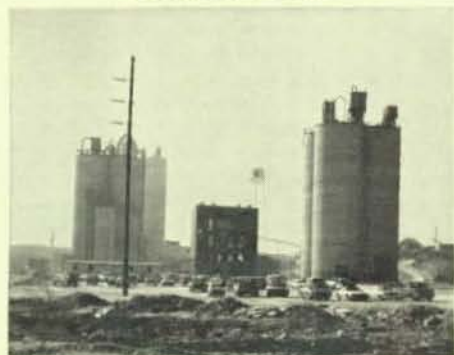
This is a view of the cement plant in Brooksville, Fla., which employs a large number of members of Local 308, St. Petersburg, Fla.
