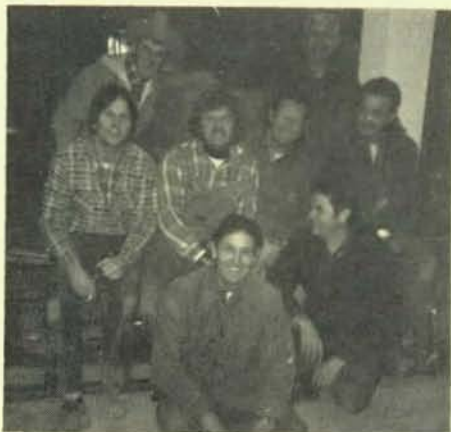
Members of Local 262, Plainfield, N.J., are shown working at the McKee building in Berkeley Heights for Liberty Electrical Corp., Bayonne, N.J. Front row, left to right, are foreman Dan Alsobrooks and Jim Moroney; second row: Paul Greaves, Richie Coddington, Jim Miller, and Andy Olexon; standing: Bob Heintz and Ted Zydiak.
