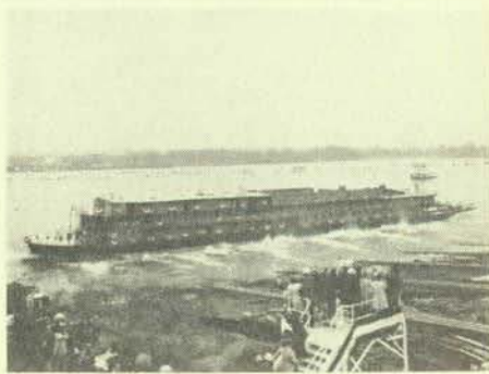
These four pictures show the various stages of construction of the steamboat Mississippi Queen at Jeff Boatworks, Jefferson, Ind. Members of Local 369, Louisville, Ky., are employed on the project.
