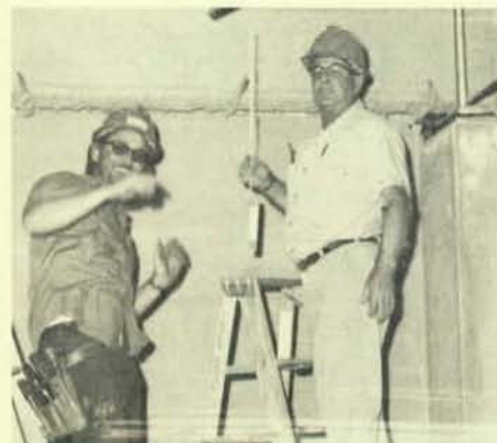
Local 130, New Orleans, La., Brothers John Ricks and John Bacques, Sr., on the Superdome job of a few years ago.
