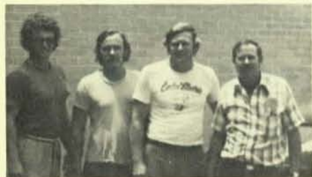
Members of the first crew working on Atlantic City's first casino, for Resorts International, are Bob Bristle, Dennis Hood, Herman Schenker, and foreman Don Tapp.
