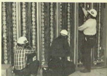
Brothers Johnny Barnes, D. L. McKee, and Glen Harrell of Local 505, Mobile, Ala., work in relay cabinets on the Degussa project for Wilson Electric Company.
