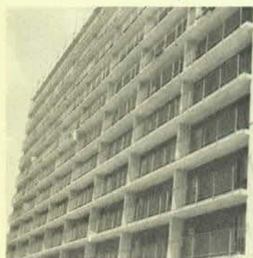
This is the modular apartment building for the elderly which is nearing completion.
