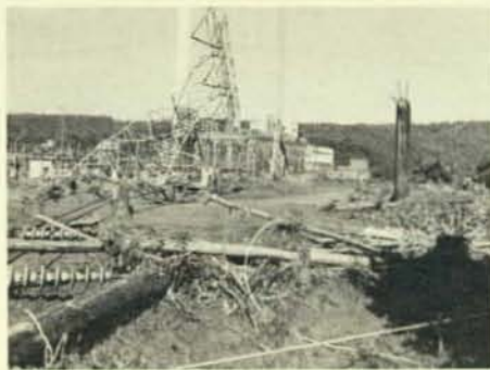
Seward Generating Station after the flood.
