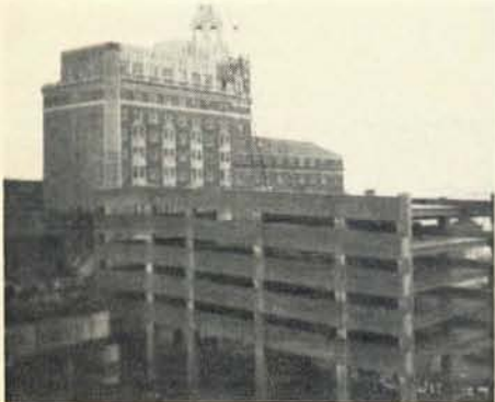
The new parking area for Caesar's Boardwalk Regency will soon be the new Benihana Hotel Casino. The aging Shelburne is in the background.
