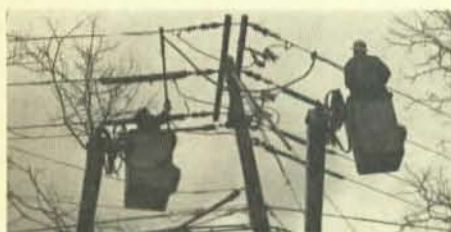
Brothers Richie Spina, left, and Bill Leggett of Local 300, Montpelier, Vt., jumping out cut-out Essex Center.
