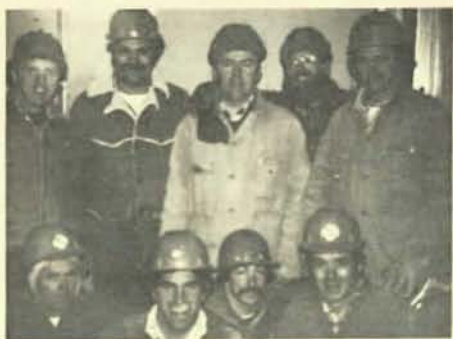
Brothers of Local 683, Columbus, Ohio, working at the Ohio Center Complex job, front row, left to right, are George Ray, Tim Keysor, Joe Caldwell and Leo Haas; back row: Sib Goelz, Kenny Tate, Terry Emrich, Denny Austin, and Dave Winters.
