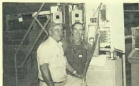
Making final terminations are foreman Mike Stathatos and Bob Shields.
