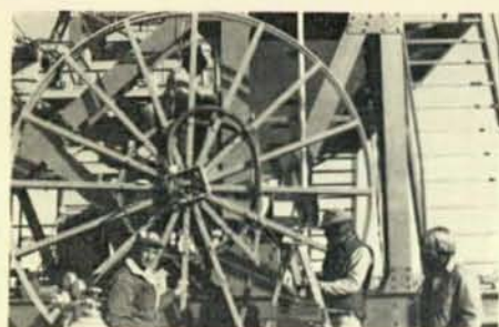
Working on the continuous pour-casting machine, left to right, are W. Carmack, C. Canella, R. King, and Rich Marchbank of Local 113, Colorado Springs, Colo.
