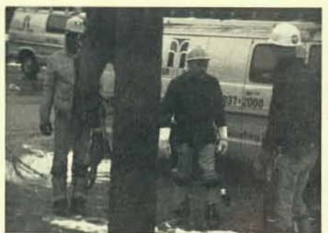
Apprentice coordinator Bob Shutter holds a pole climbing seminar at Courier Cable.
