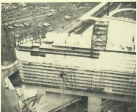
The Hyatt-Regency Hotel job under construction.
