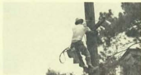
A Local 398 lineman is shown at work.
