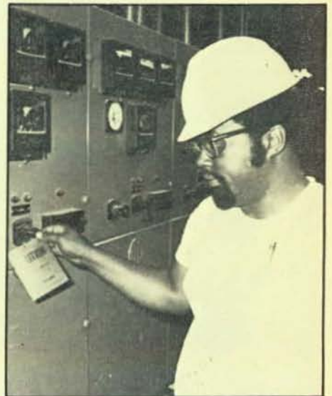
LU 2337 member Leon Preston, equipment operator, tags out a piece of equipment at the Big Brown facility.
