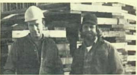
Erwin Mize and Jimmy Coker are employed by Price-Fewell Electric Company and are working on the addition to the State Revenue Department Building.
