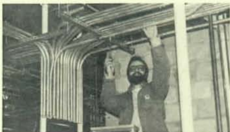
Joe Marricco lines up conduit on telephone rack.
