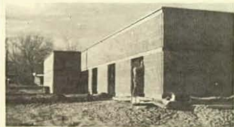
This is looking northeast at the new building.
