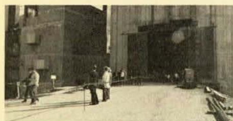
Members of Local 369, Louisville, Ky., show their families "The Big Job"—The Marble Hill Nuclear Generating Station.
