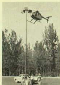
Members of Local 728, Ft. Lauderdale, Fla., employed by E.C. Ernst, set light poles at the Coral Square Shopping Center in Coral Springs.
