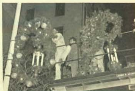
Local 271, Wichita, Kans., members installed the downtown Christmas decorations. Here, Brother Mike Killian supervises as Brothers Carl Lambert and Rick Gilbert hand a post fixture from a manlift.
