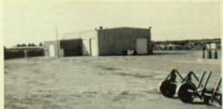
Site of the new warehouse in Manteca.
