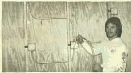
Apprentice Dean Connor, Local 640, Phoenix, Ariz., shows the art of pulling wire as he demonstrates to other apprentices at the JATC.
