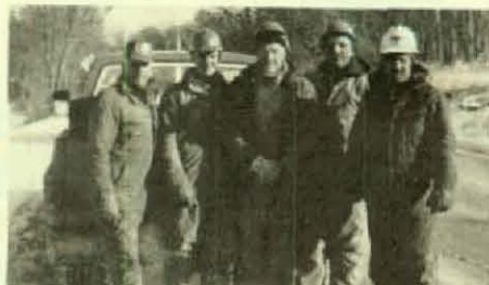
Pictured is the L. E. Myers crew on 138-KV line in Oglesby, Illinois. Left to right are Brothers Bob Erickson, Bob Christa, Rod Johnson, Jim Carlock and Dan Mahnke.
