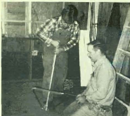
Journeyman Richard Hanson (kneeling) instructs apprentice Dave Dryer in the finer points of pipe bending.
