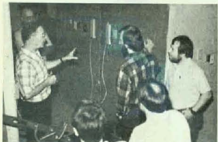
Instructor Pete Webb briefs the journeymen on troubleshooting telephone equipment. (Photos submitted by Local 666, Richmond, Va.)
