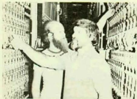
Benji Durham, left, and Willie Evans take a last look at the electromechanical step switches. The new GTD No. 5 electronic digital switch is in and working. It is positioned just to the left, but not visible in picture. (Photo submitted by Local 289, Durham, N.C.)
