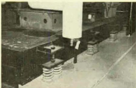
A unique aspect of the project is the free-standing generator bases poured with a mixture of concrete and punched-metal pellets to absorb full running vibration. (Photos submitted by Local 1, St. Louis, Mo.)
