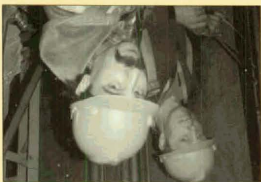
Local 246, Shubenville, OH, Bros. Randy Truax and Tim Corona of work on the Cardinal Power Plant "stack" job.
