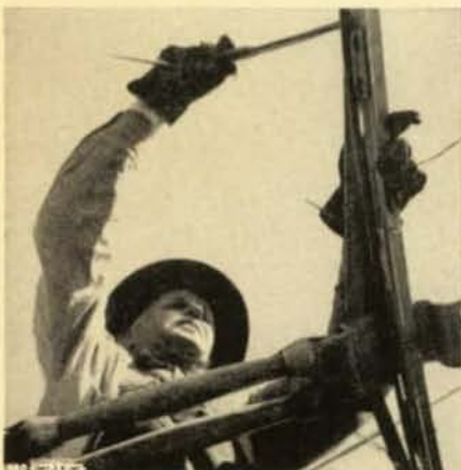
Member: Leslie Hurd installs curve segment in overhead trolley system on the busy Mission-Van Ness line.
