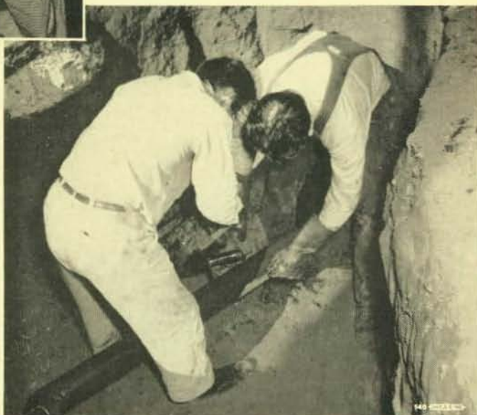
Below: Pipe wrappers John Moore and Joe Hughes of L.U. 1245, use proper safety equipment in applying tar at new section of gas main.
