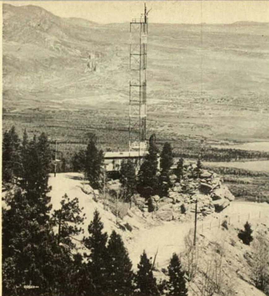
The summit transmitter site of the National Bureau of Standards radio propagation field station at Cheyenne Mountain, Colorado. The station is located on top of a mountain 9,000 feet above sea level and commands a radio view that is comparatively flat for about 300 miles in easterly direction.
