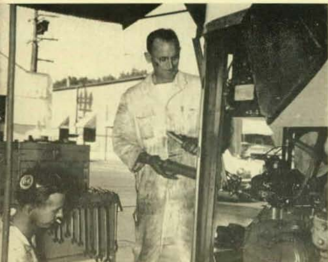
Above: George Smith and Verne Flannery of L.U. 1245 overhaul the engine of a motor coach of the Sacramento City Bus Line, where they work as mechanics.
