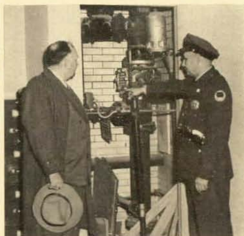
Below: Chief Guard Victor Kruge, right shows Ed Redemeier a typical sprinkler alarm enclosure, made by the Potter Co.
