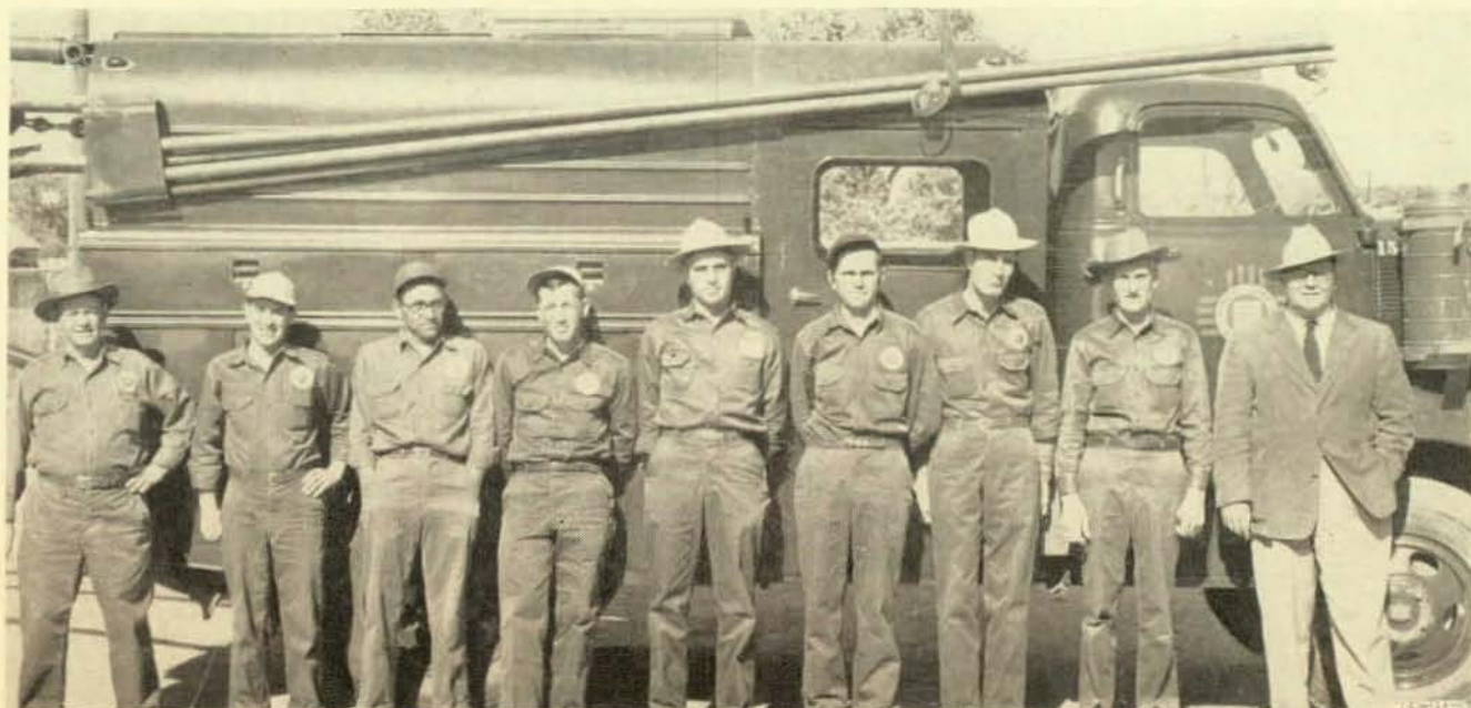
This group of members of L. U. 611, Albuquerque, N. M., comprising the Belen line crew of the Deming Power Plant of the Public Service Company, has been credited with being the most efficient crew in the entire organization. From left to right are shown: Jose Garcia, utility worker; Andy Aragon, Class A helper; Manuel Bibiano, third year apprentice lineman; Gene Foster, truck driver; Russell Hendren, utility worker; Ray Theiler, lineman; Sam Chavez, lineman; Joe Nugent, line foreman, and K. L. Bradshaw, superintendent.
