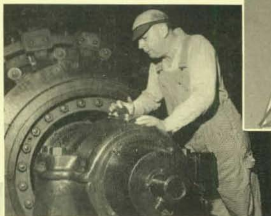
Right: L. G. Glas-son, Recording Secretary of L.U. 1245 checks oil rings of converter at substation.
