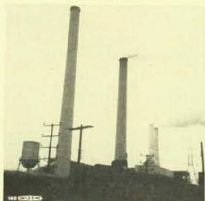
Power plant at W. Broad and River Streets. At far right is the new addition put in operation early in 1955.
