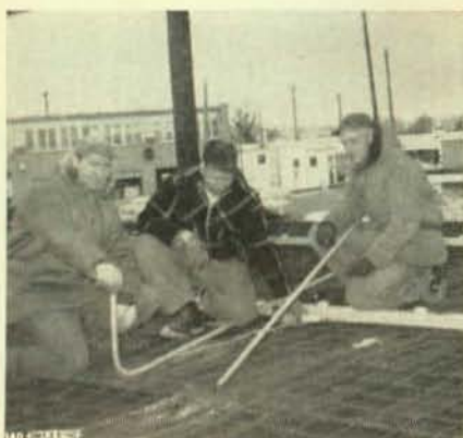
Electricians of Central Electric Co., Minneapolis, at the Richfield State Bank, installing Howard Phone Duct and Low Floor Outlets. The men, members of Local 292, are Merle Kolbe and Evert Erickson. The third man is unidentified. At right: Merle Kolbe checks Howard Phone Duct and PBX Location.
