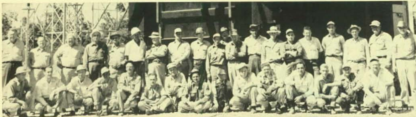
These members of Local 702, West Frankfort, Ill., are a number of traveling members employed on construction of the Joppa Steam Electric Plant nearby.
