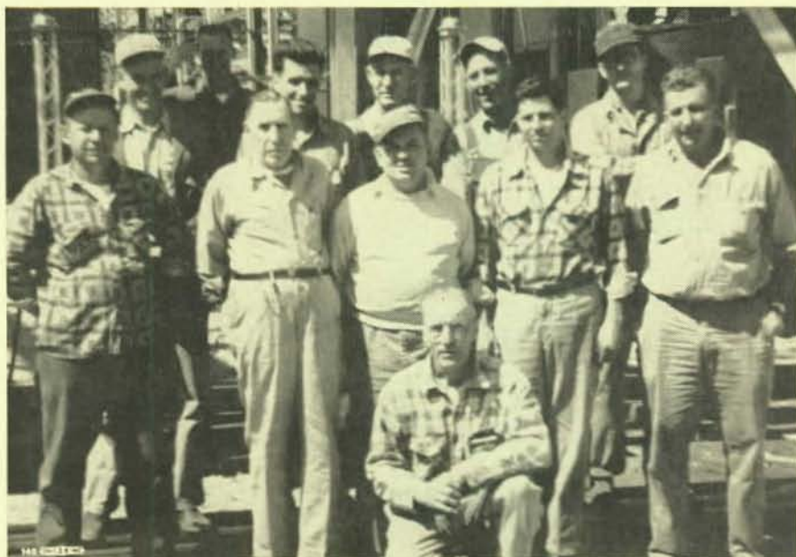
Local 160 and Local 292 crew who completed the Southtown Substation erection. Dewey Anderson, foreman, in front. Next row, left to right: John Ellis; Ed Bantle; Bill Leeper; Dale Leigh, and Clarence Graeber. Back row: Clarence Anderson; Roy Severson; Don Mason; Irving St. John; Robert Gelina, and Mike Conway.
