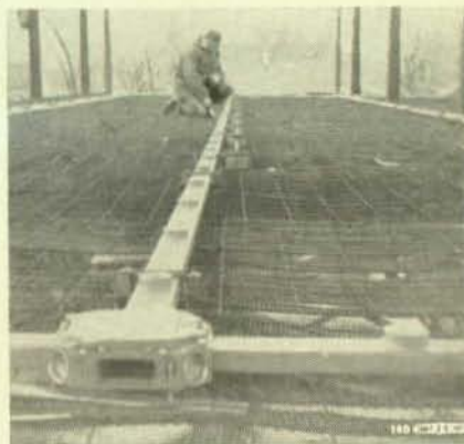
Electricians of Central Electric Co., Minneapolis, at the Richfield State Bank, installing Howard Phone Duct and Low Floor Outlets. The men, members of Local 292, are Merle Kolbe and Evert Erickson. The third man is unidentified. At right: Merle Kolbe checks Howard Phone Duct and PBX Location.
