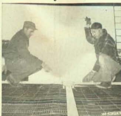
Electricians of Central Electric Co., Minneapolis, at the Richfield State Bank, installing Howard Phone Duct and Low Floor Outlets. The men, members of Local 292, are Merle Kolbe and Evert Erickson. The third man is unidentified. At right: Merle Kolbe checks Howard Phone Duct and PBX Location.
