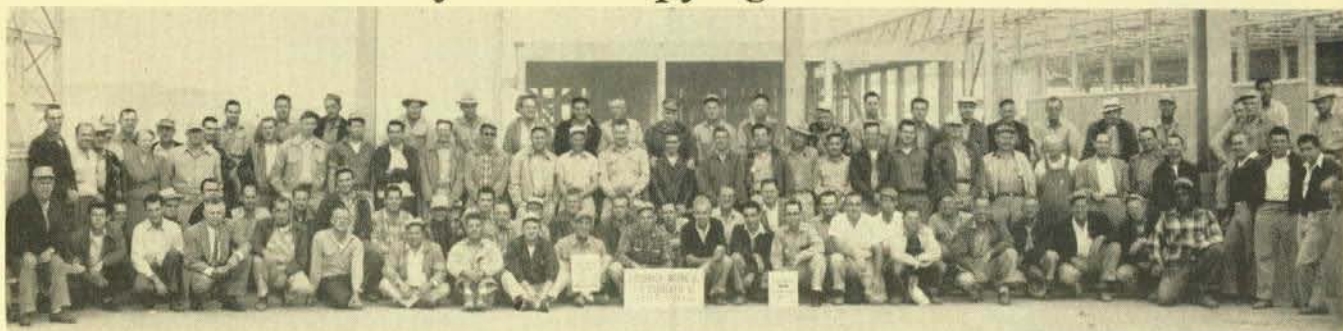
Members of Local 11, Los Angeles, Calif., pose before the site of the new Ford-Mercury plant under construction in Rivera, Calif.
