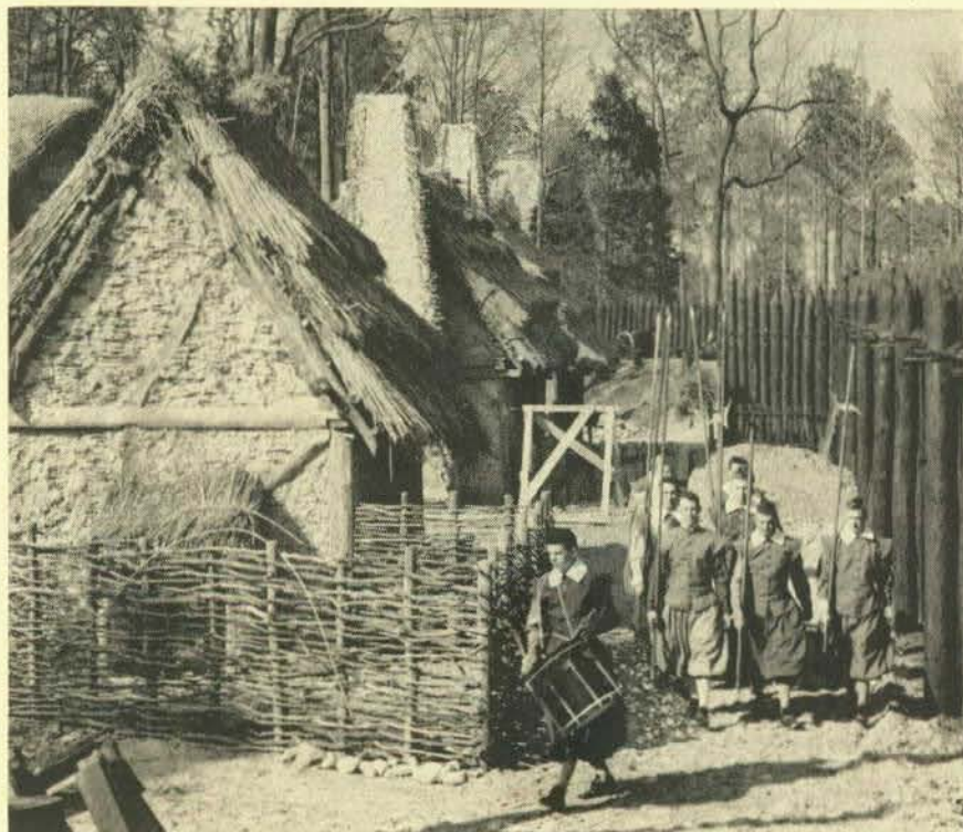
Inside the reconstructed James Fort, Jamestown, Va. Electrical installations at the Jamestown Exposition and other attractions in the area were made by members of the Richmond, Newport News, and Norfolk locals.
