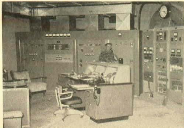
Left: Exterior view of the building housing radio-transmitting equipment of C.F.C.F. installed by members of Local 568, Montreal, near Caughnawaga on the Indian Reserve. Right: Interior view of the radio-transmitters and station equipment being installed. The building has its own power plant and all the equipment is completely automatic.
