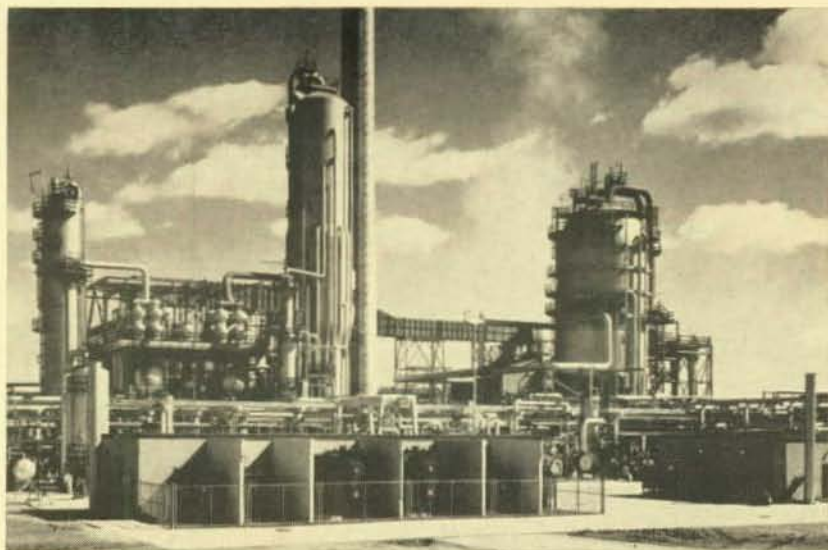
One of 13 switch-houses, this unit houses gear for unit behind it. Two transformers are 5000/6250 KVA; rated voltage 13.8 KV to 2.4 KV; two others are 750 KVA with voltage from 13.8 to 480.
