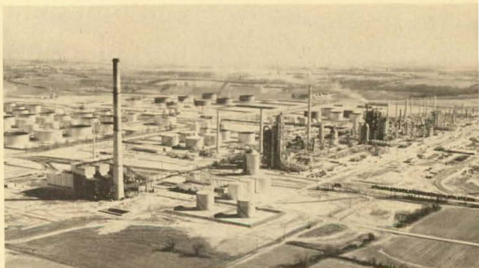
Aerial view of the world's largest oil refinery operated by the Tidewater Oil Co., Tidewater, Delaware, near Wilmington. Power station building with 500-foot stack can be seen left foreground.
