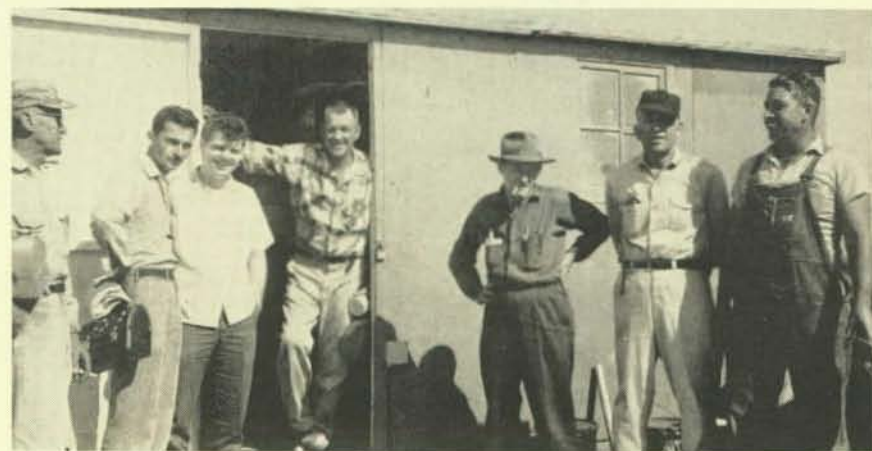
These men are finding many interesting aspects in the work they are doing on a new Safeway warehouse and distribution center in Martinez, Calif. Their names and fuller details are in the letter of Local 302.
